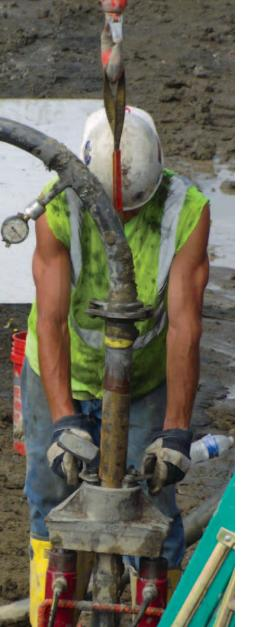
Geotech Services was called in by E.S. Wagner of Toledo (the general contractor on the job) to do the compaction grouting beneath the new sidings prior to the track bed and rail installation to help stabilization. The goal was to get ahead of
